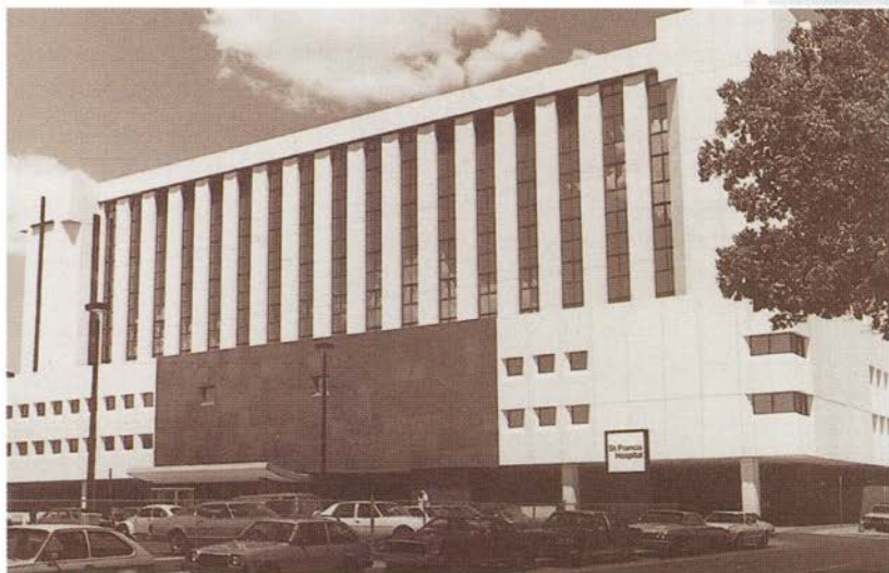
View of the 1978 addition to St. Francis Hospital, Wichita.
