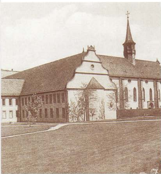
Former convent of Himmelspforten, Würzburg, now a diocesan retreat house. (building at left)
